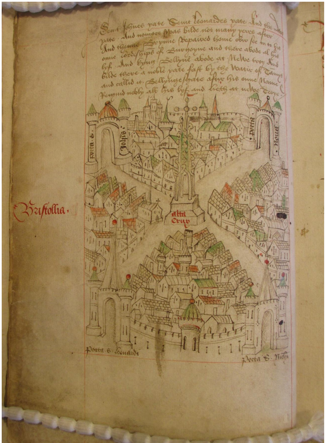
Bristol Archives, CC/2/7, f. 5v, drawing of the city in the Bristol Kalendar. With the kind permission of Bristol Archives.
